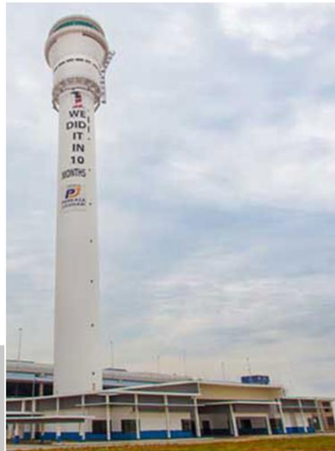
The tallest ATC tower (141.9 m)
